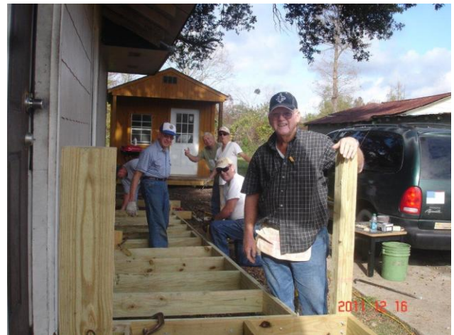
Starting to shape up and look like a ramp
