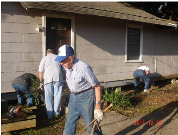
First things first. Demo and clean up.
