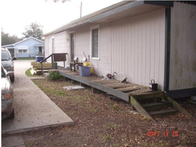
The old ramp to be replaced. Let's get started.
